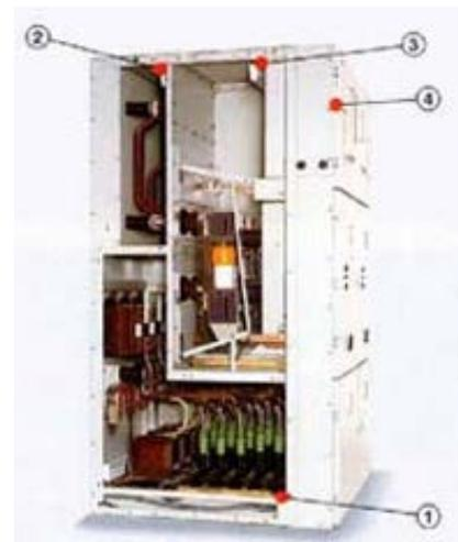
1. Sensor in outgoing cable compartment
